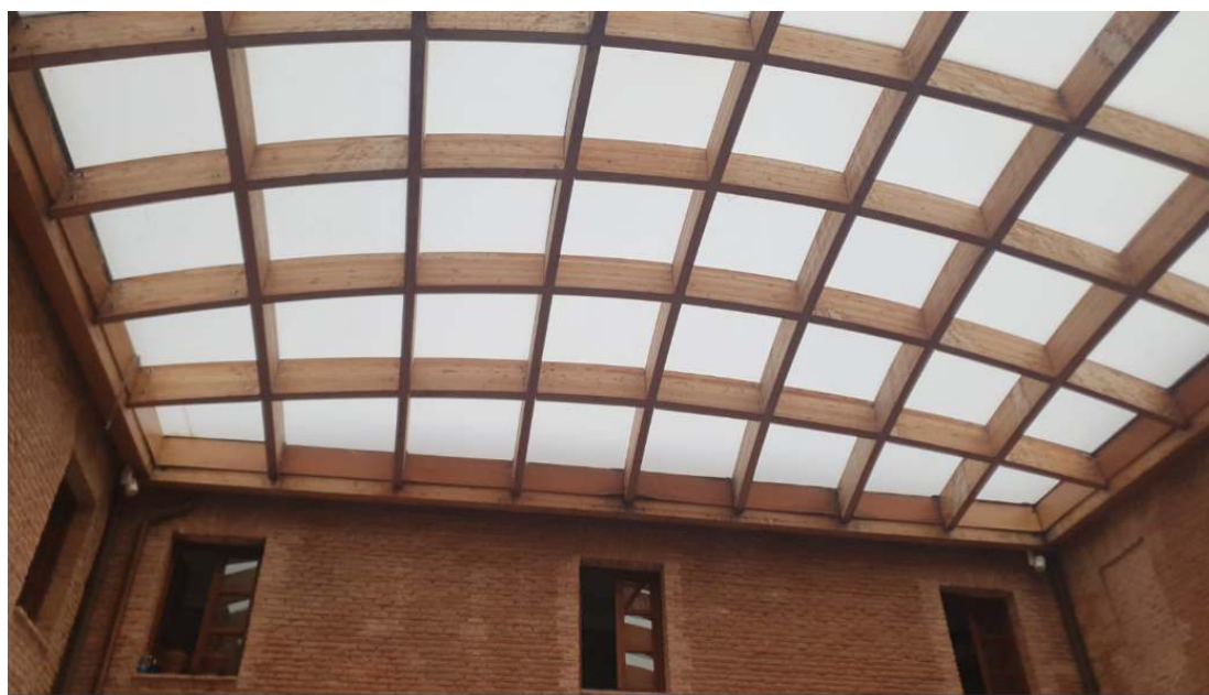
Lucernario a rehabilitar
