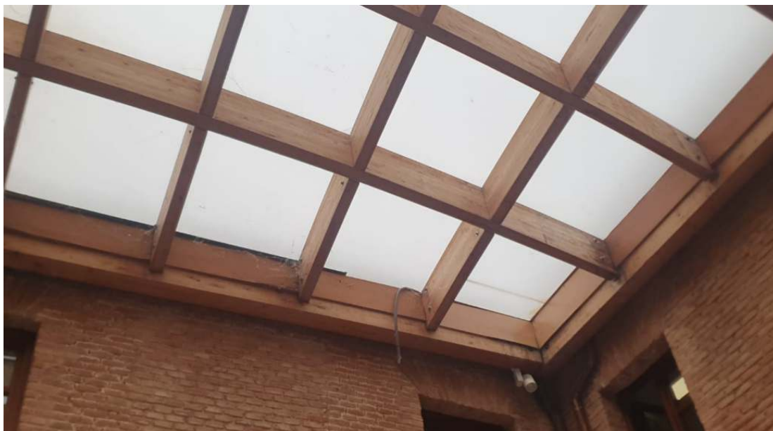
Lucernario a rehabilitar
