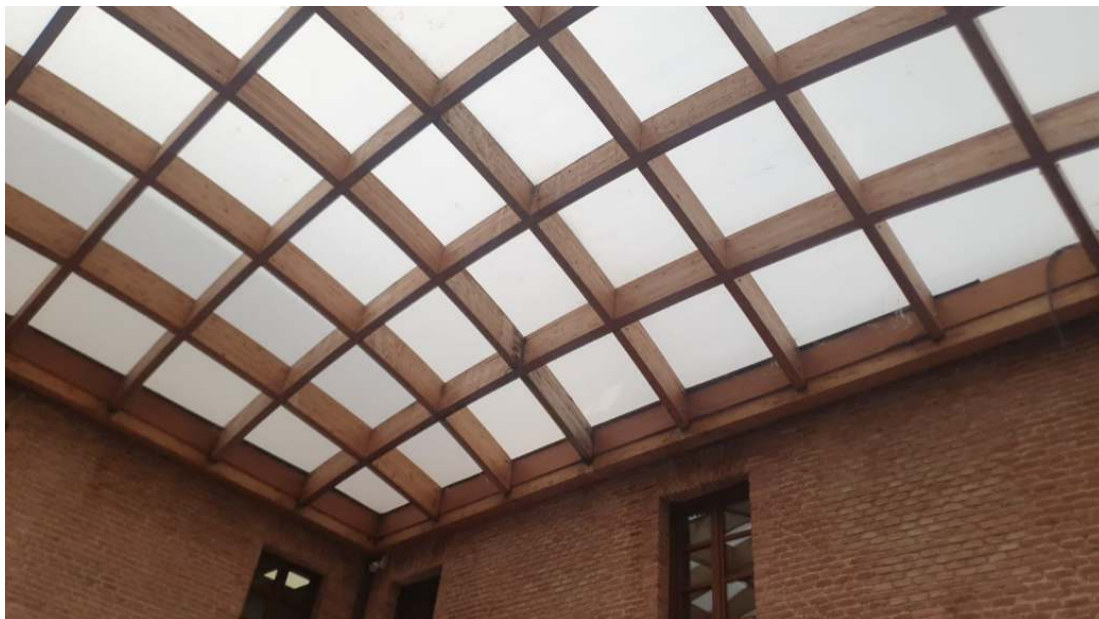
Lucernario a rehabilitar
